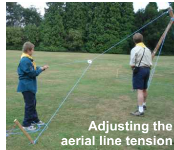
Simple sheer legs. Note the guide for the aerial line
